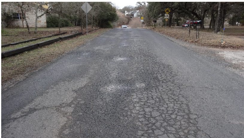
Figure 1: Alligator Cracks
